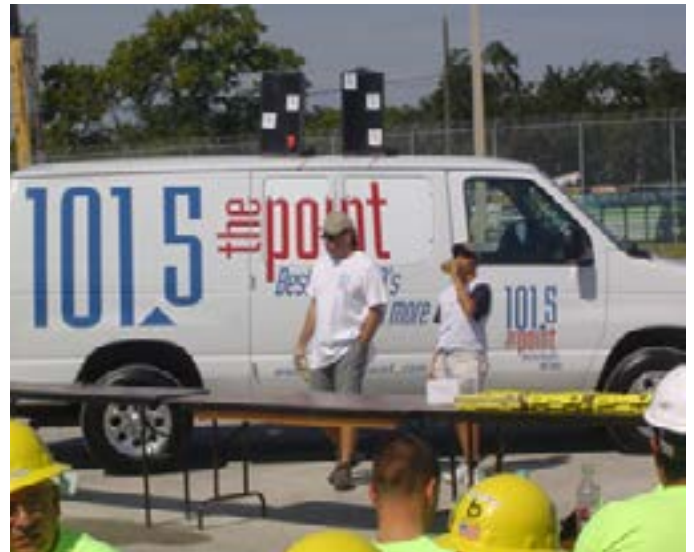
Think about inviting a local radio station to your jobsite. The radio personalities will lighten up the day and provide music throughout the days activities.
